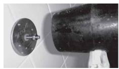
14. Verify the length of the nut from the *WingIt*<sup>TM</sup> faceplate is correct (step 8) – Then hit the *WingIt*<sup>TM</sup> firmly with a rubber hammer.
